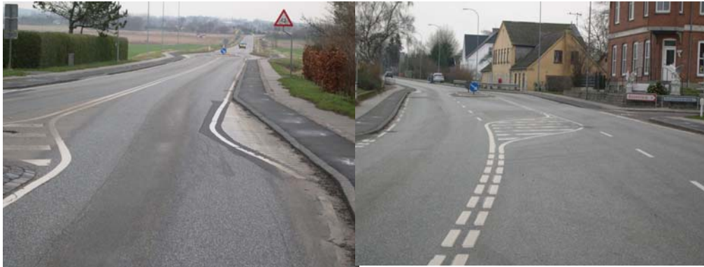
Figure. 14. Pictures from one of the through-roads in a town called Stenmangle, 10 years after construction.
